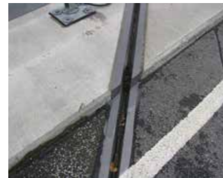
Flush-mounted steel profile in the walkway
