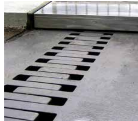
Finger-type expansion joint with stainless steel walkway
