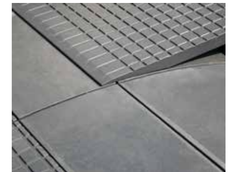
Surface detail of roller shutter joint
