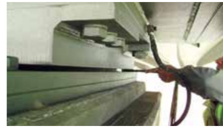
Installation of a fixed restraint device
