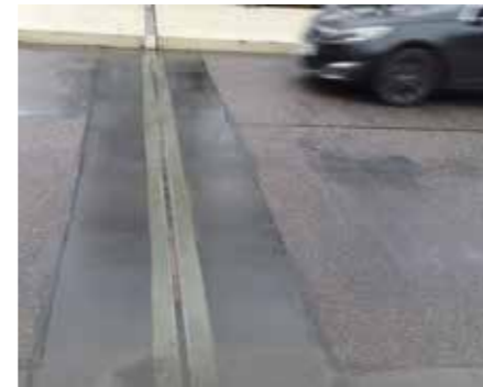
Single gap expansion joint
