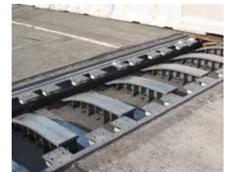
Roller shutter joint during installation
